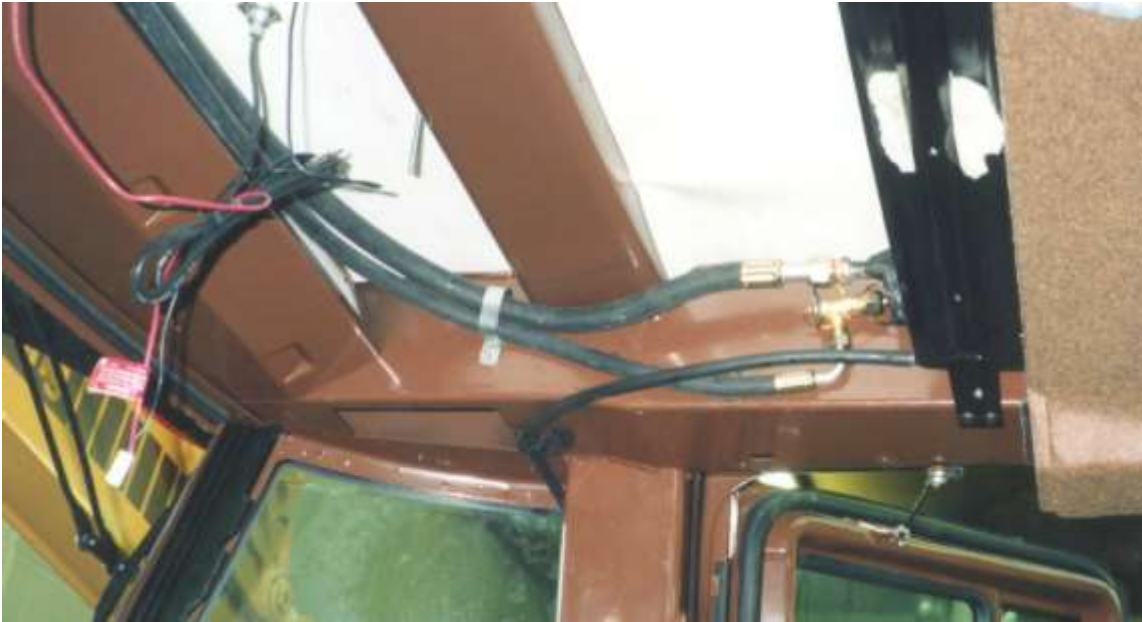
Evaporator and drain pan in place with hoses and drain tubes.
