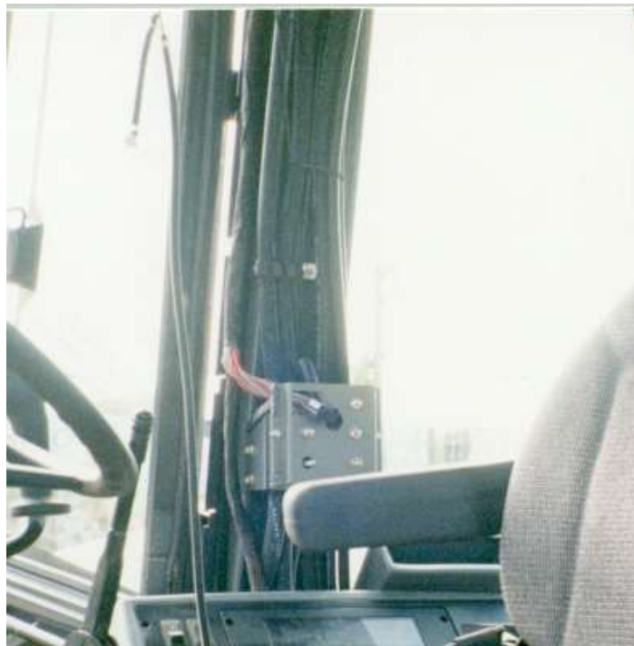
Hoses running up column on right side of cab.
